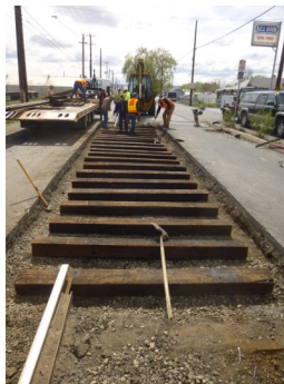
River Road track repair in progress
